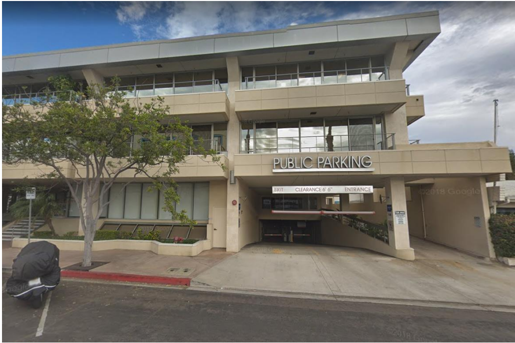
Parking Entrance 7777 Fay Avenue
